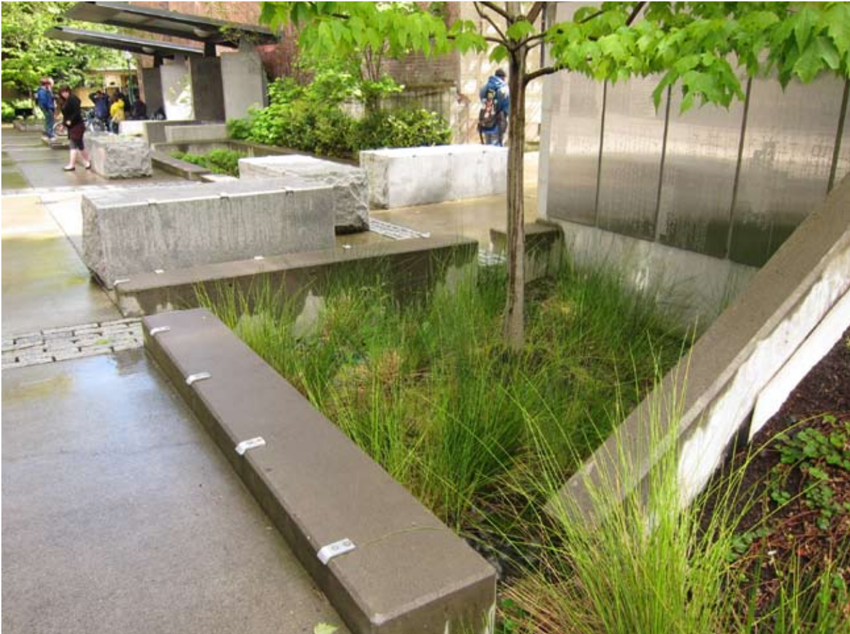
Artful Infiltration Basin for impervious areas in Portland, OR, U.S.A. (Photo by Author)
