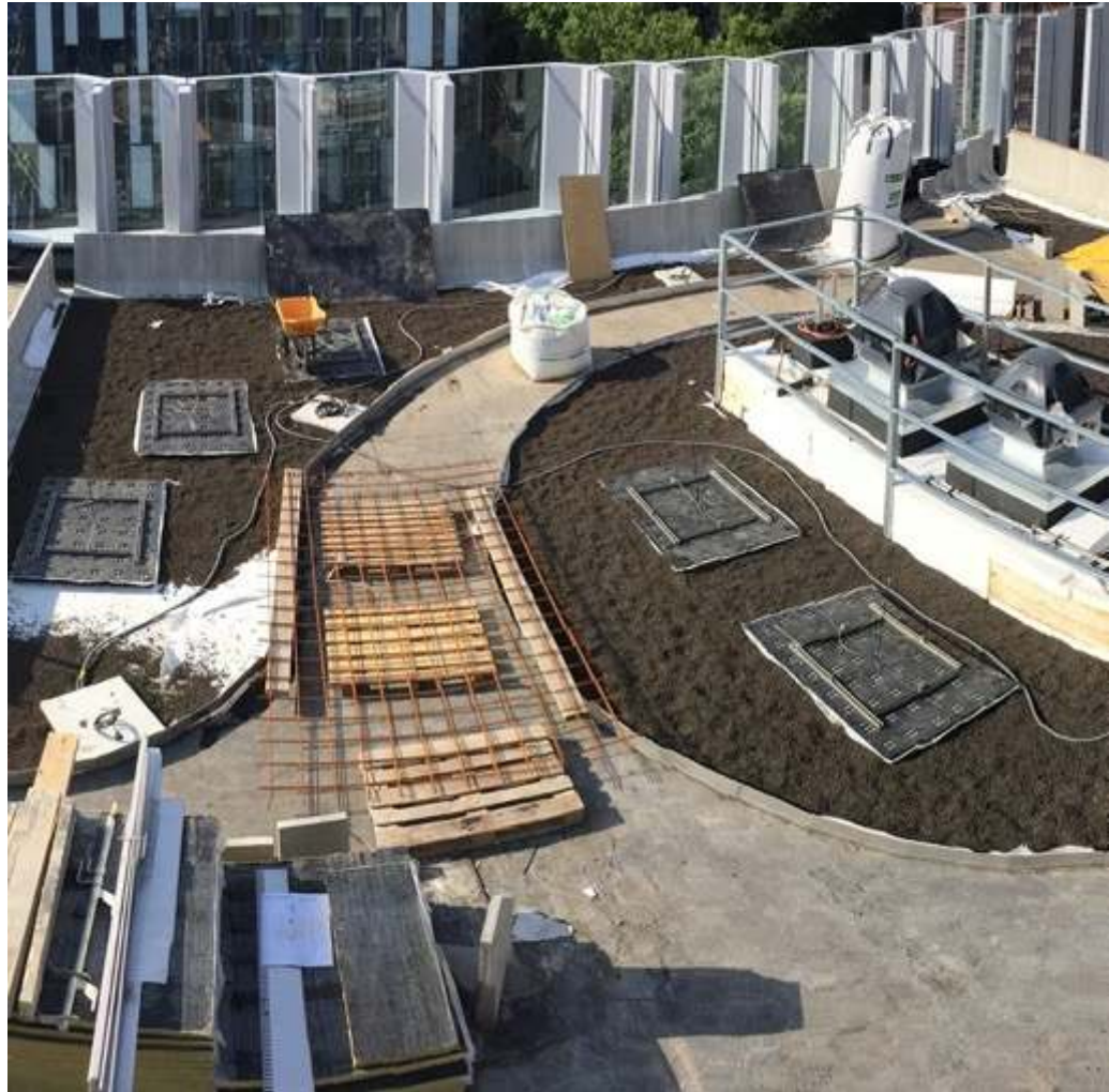
“Oasis system” (50L/m 2 ) + dripline irrigation
