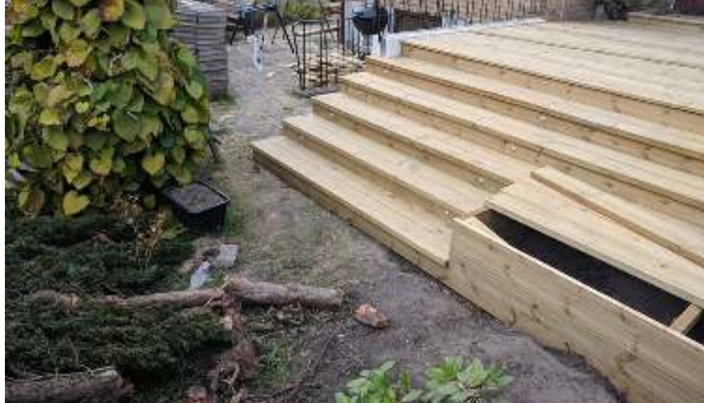
Housing improvements such as decks and patios have been recognized as a major source of tree decline in some cases. Unsurprisingly, most of these adaptations happen when property changes hands.
